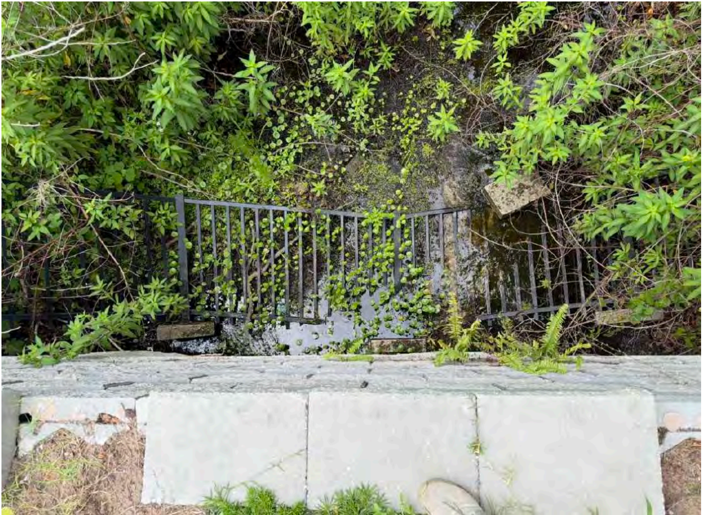
2 2-Fence Removal Date Taken: 6/10/2026 Taken By: URS
